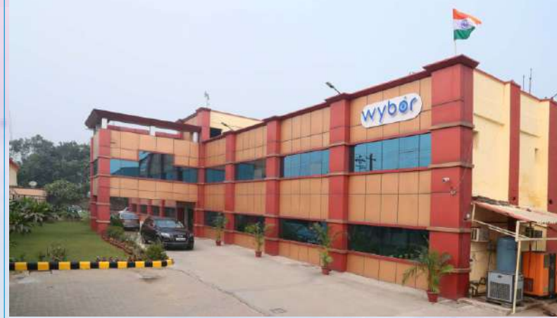
AIR CONDITIONER PLANT
